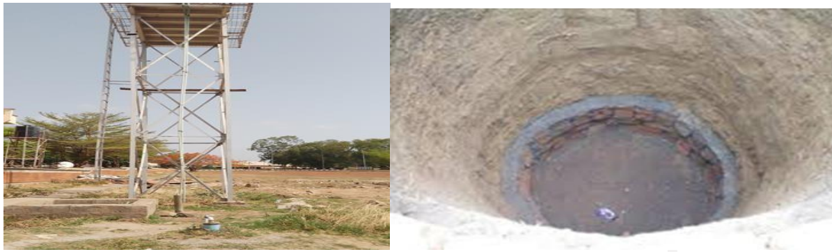
Figure 2. Borehole and Hand-dug well
