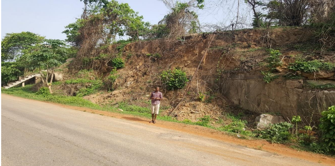
Plate 1: Road Section Showing Fresh Rock Buried under Weathered Regolith
