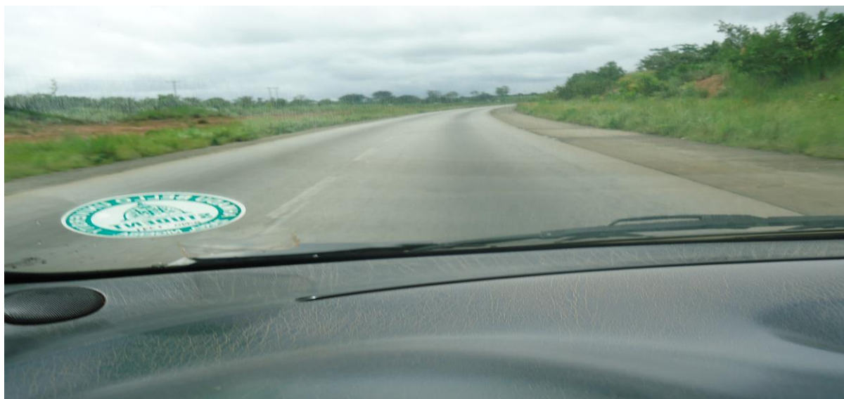
Plate 4: Sharp bend at Konar Bature along Kaduna-Abuja Road
