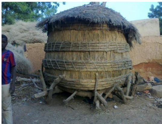
Figure 3: Thatched Silos at Yardaji
