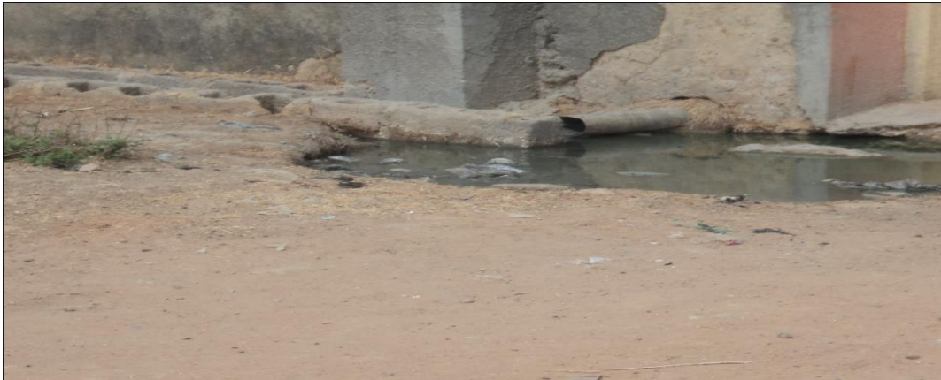
Fig. 7: A house where the domestic waste and bath effluent to flow on to the street in Dogarawa
