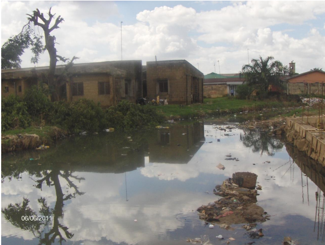
Plate 2 Buildings on Flood- Prone Area in Kabala Costain, Kaduna. These buildings are on a floodplain and therefore, experience flooding at the slightest increase in rainfall
