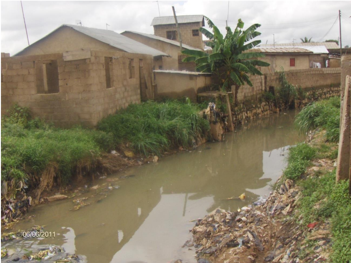
Plate 1 Building on Flood prone Area in Nassarawa, Kaduna These houses are on a floodplain and are consequently at the mercy of flooding whenever rainfall increases.
