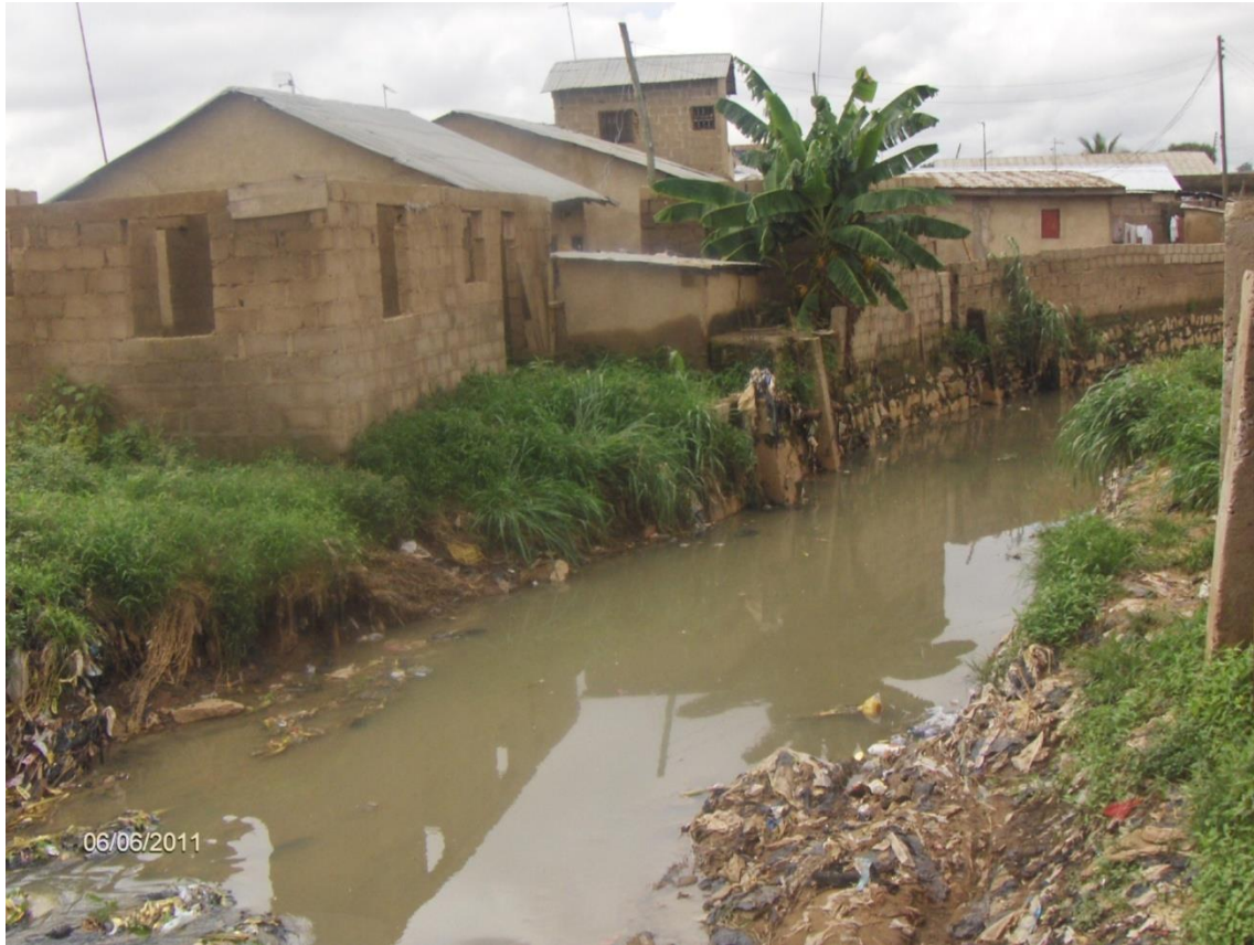
Plate 1 Building on Flood prone Area in Nassarawa, Kaduna These houses are on a floodplain and are consequently at the mercy of flooding whenever rainfall increases.
