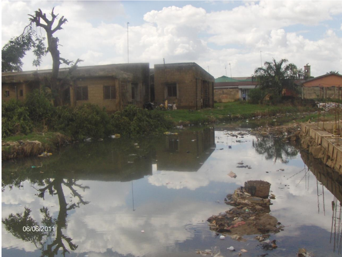
Plate 2 Buildings on Flood- Prone Area in Kabala Costain, Kaduna. These buildings are on a floodplain and therefore, experience flooding at the slightest increase in rainfall
