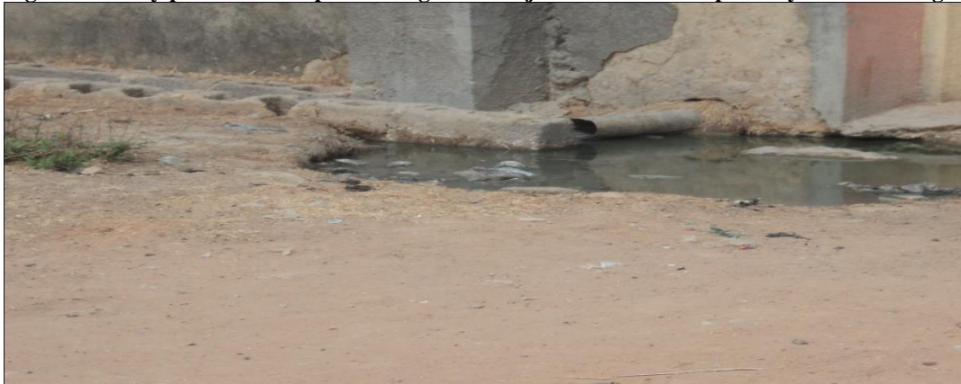
Fig. 6: A house where the domestic waste and bath effluent to flow on to the street in Dogarawa
